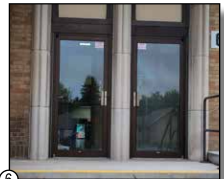
⑥ HOLLOW METAL DOORS & HOLLOW METAL FRAME
