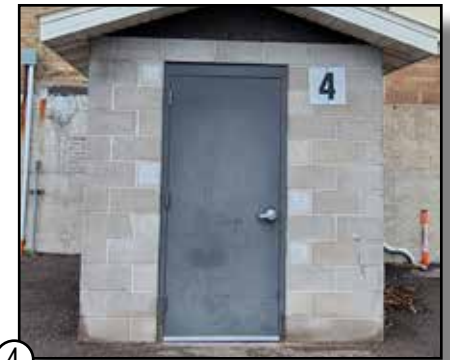
④ HOLLOW METAL DOORS & HOLLOW METAL FRAME
