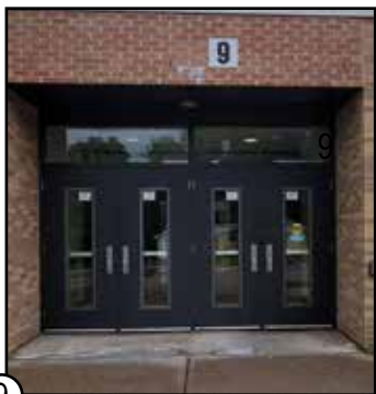
⑨ HOLLOW METAL DOORS & HOLLOW METAL FRAME
