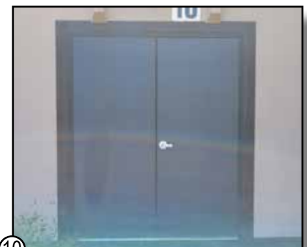
10 FRP DOORS & HOLLOW METAL FRAME
