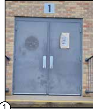
① HOLLOW METAL DOORS & HOLLOW METAL FRAME
